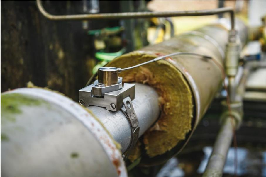
Wi-Corr® Clamp is a revolutionary wireless monitoring system. Through a self-organising network of permanently or temporarily installed, wireless enabled sensors, accurate pipe wall thickness and temperature can be obtained cost-effectively, enabling corrosion and erosion to be precisely monitored. This information allows a proactive approach in planning of turnarounds and preventative action.
